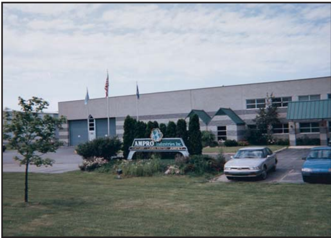
Front of Ampro building looking north.
